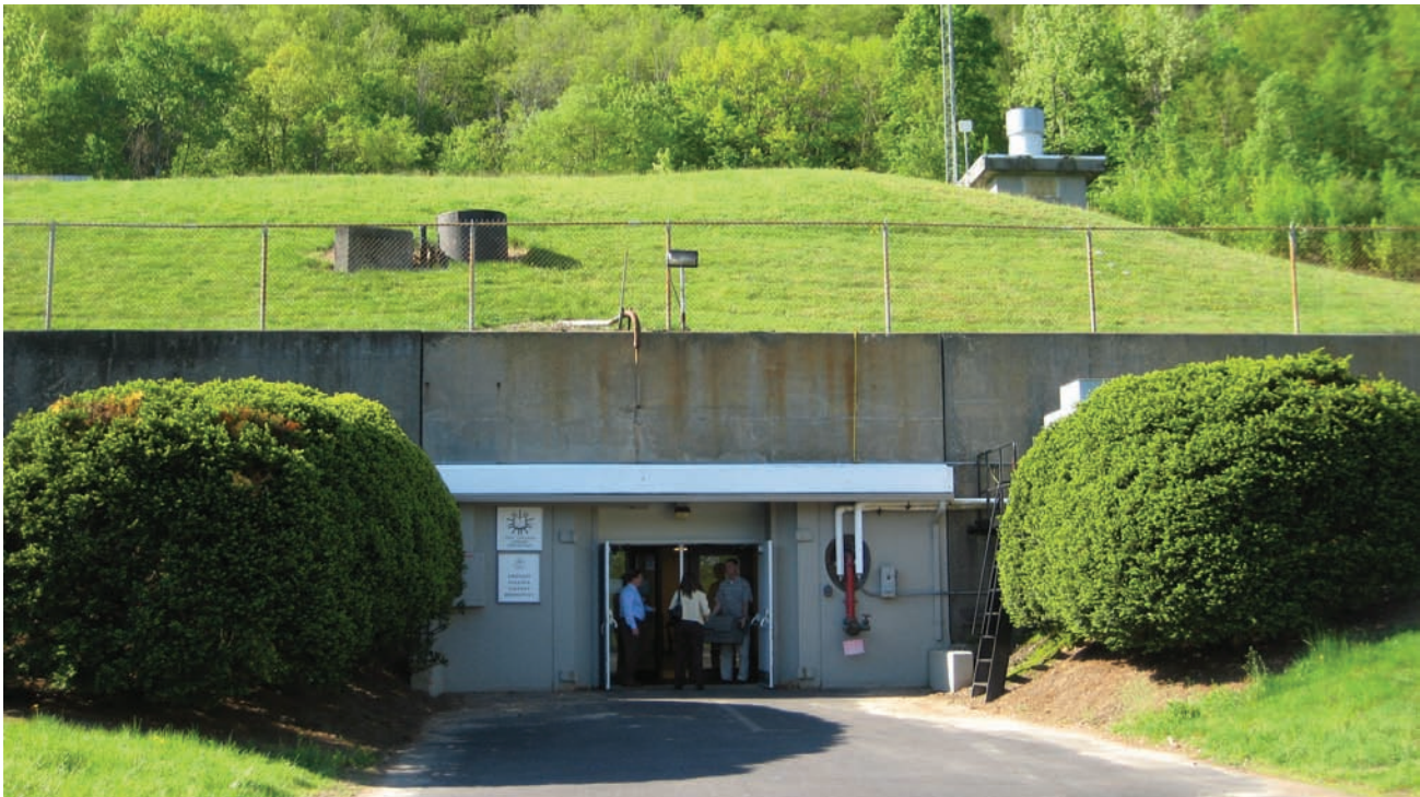
Five College Depository
